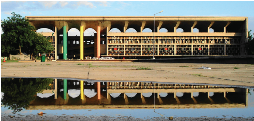
10 The High Court is equipped with a double roof that encloses the entire building in its shade.
