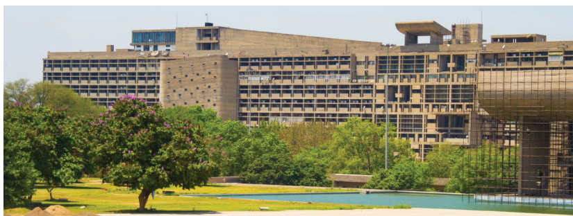
The 240m high Secretariat was the tallest building in Punjab when it was built.
