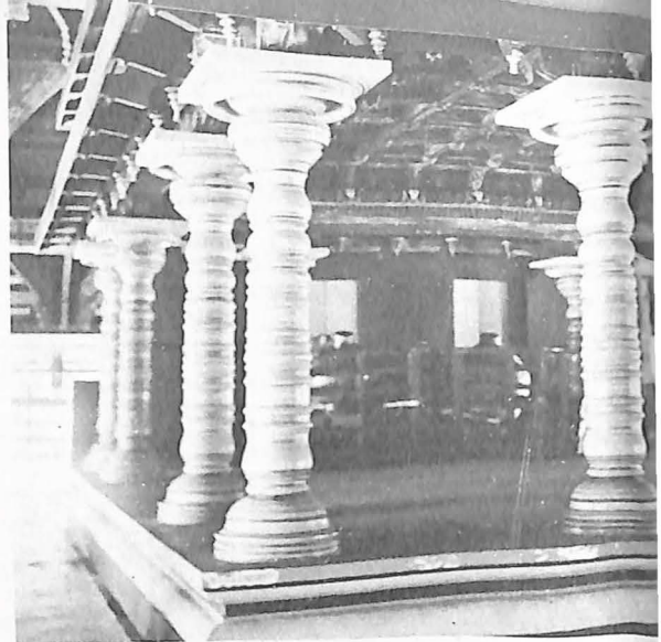
The extension of the stage (between two of the corner pillars of the stage plinth) of the Vadakkunnathan Kuttambalam as seen from the stage front. Perhaps remnants of the mattavarani-s .
