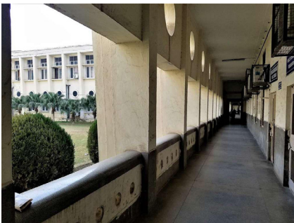
Main corridor of the Government Medical College, Patiala. Picture Credits: Wikimedia Commons.
