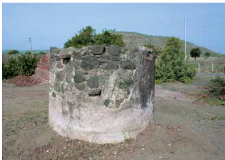
4 Remains of the monitoring tower for the underground channel at Khuldabad.
