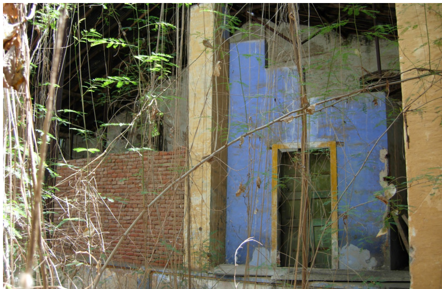
Last remaining sections of the Gaebele Theatre. Photo by Gobi G.
