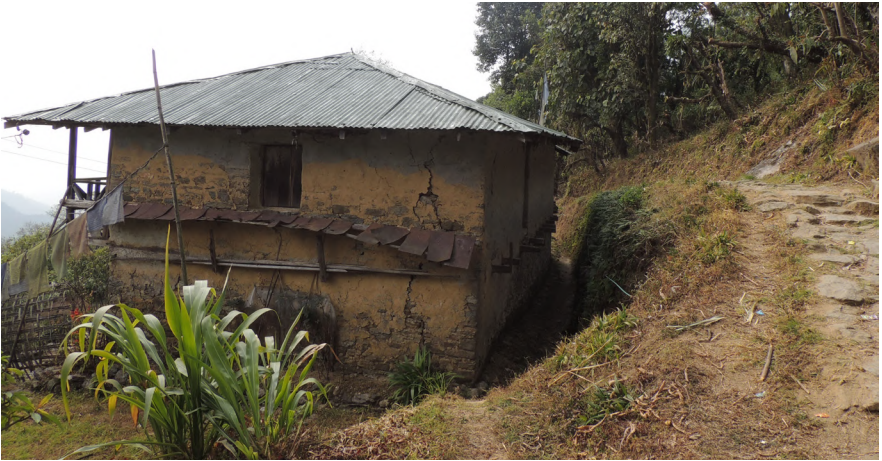
An old house made of mud, wood, and ikra style at Yalli village. Photo by Martin Sada.
