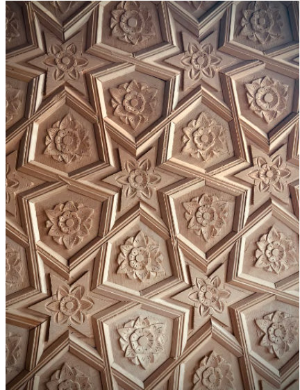
Khatambandh —intricate hand-crafted wood paneling in traditional Kashmiri architecture. Photo by Syed Muneeb Masoodi.
