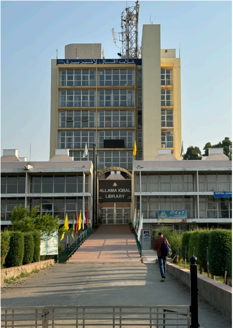
Allama Iqbal Library, Shivnath Prasad's modernist vision in concrete and light. Photo by Sheikh Intekhab Alam.
