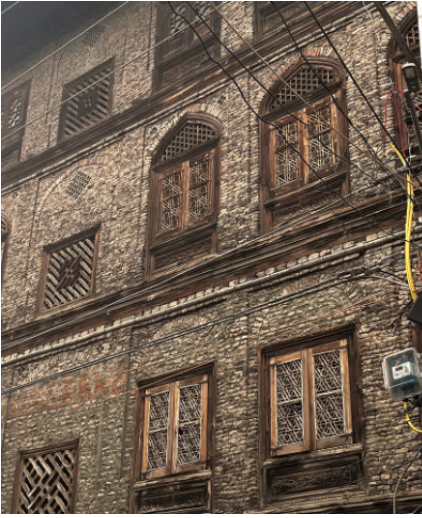
Dhajji dewari —traditional Kashmiri houses with timber-brick lattice framework. Photo by Taha Mughal.
