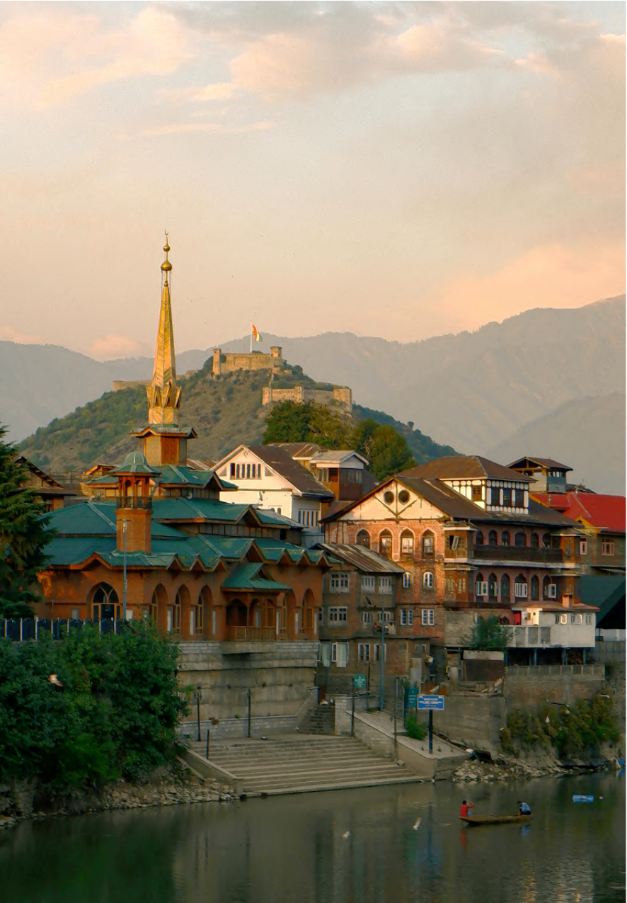
Dhajji dewari -style heritage buildings in Srinagar. Picture Credits: Sheikh Basim/Pexels.
