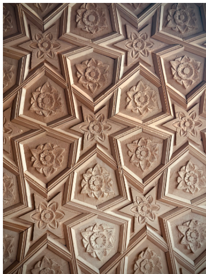
Khatambandh —intricate hand-crafted wood paneling in traditional Kashmiri architecture. Photo by Syed Muneeb Masoodi.
